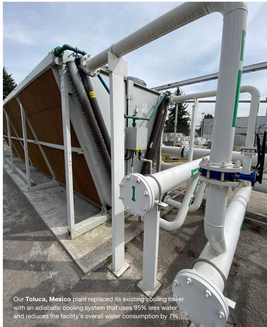
Our **Toluca, Mexico** plant replaced its existing cooling tower with an adiabatic cooling system that uses 95% less water and reduces the facility's overall water consumption by 7%.
